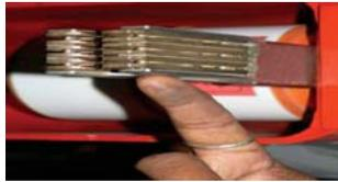
**Insulators:** The presence of contaminants on high voltage insulators made of ceramics, epoxy and Teflon can cause dielectric breakdown and arcing between otherwise non-conductive surfaces (commonly known as tracking). The result is expensive equipment damage and power outages. Thus periodical cleaning is a requirement in all high voltage applications in power generation units, distribution substations and transmission lines.
